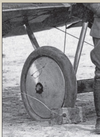
Undercarriage detail from the unidentified OAW built Albatros D.Va shown on page 6. Note the OAW style of tyre valve access cover D13.
